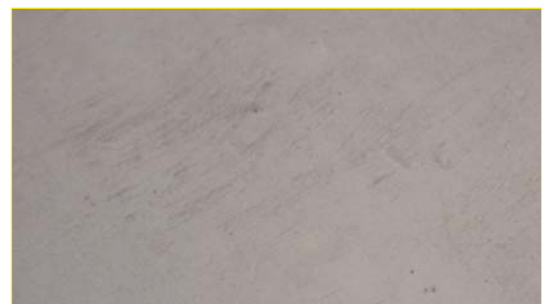
Steel Trowel Finish
